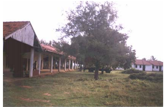
Repairs to the Grace Church Care Center
